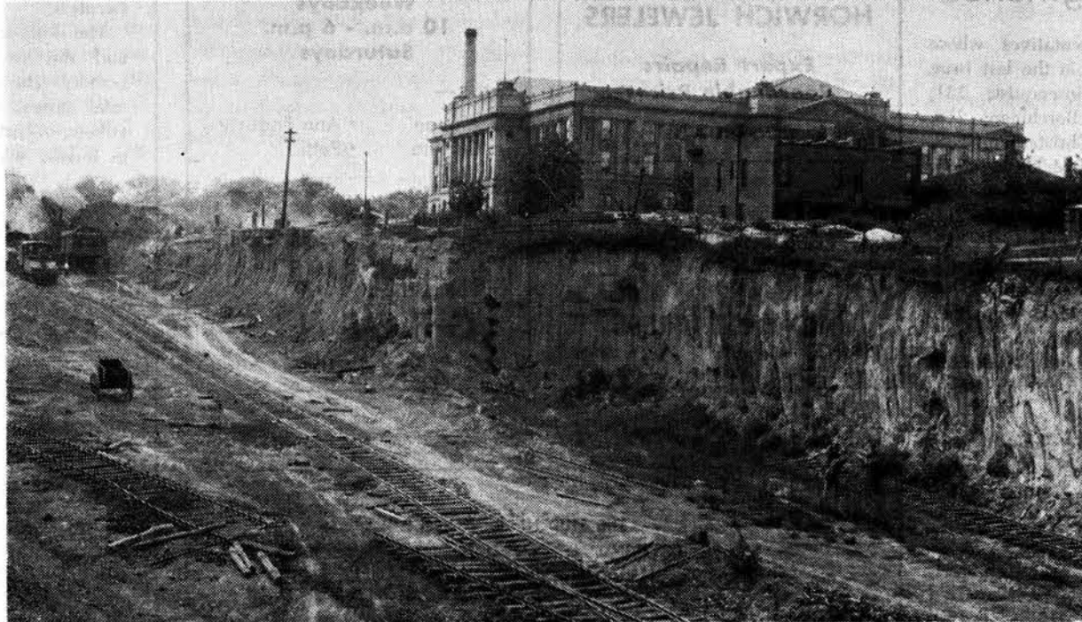
Top: Central High school in 1918 prior to lowering of Dodge Street hill. Bottom: Central during reconstruction of Dodge Street.
