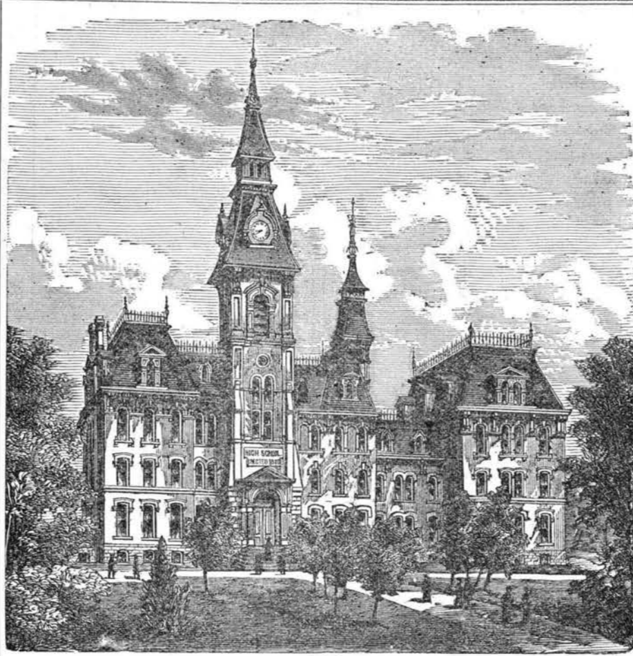
View of the Omaha High School Building.
