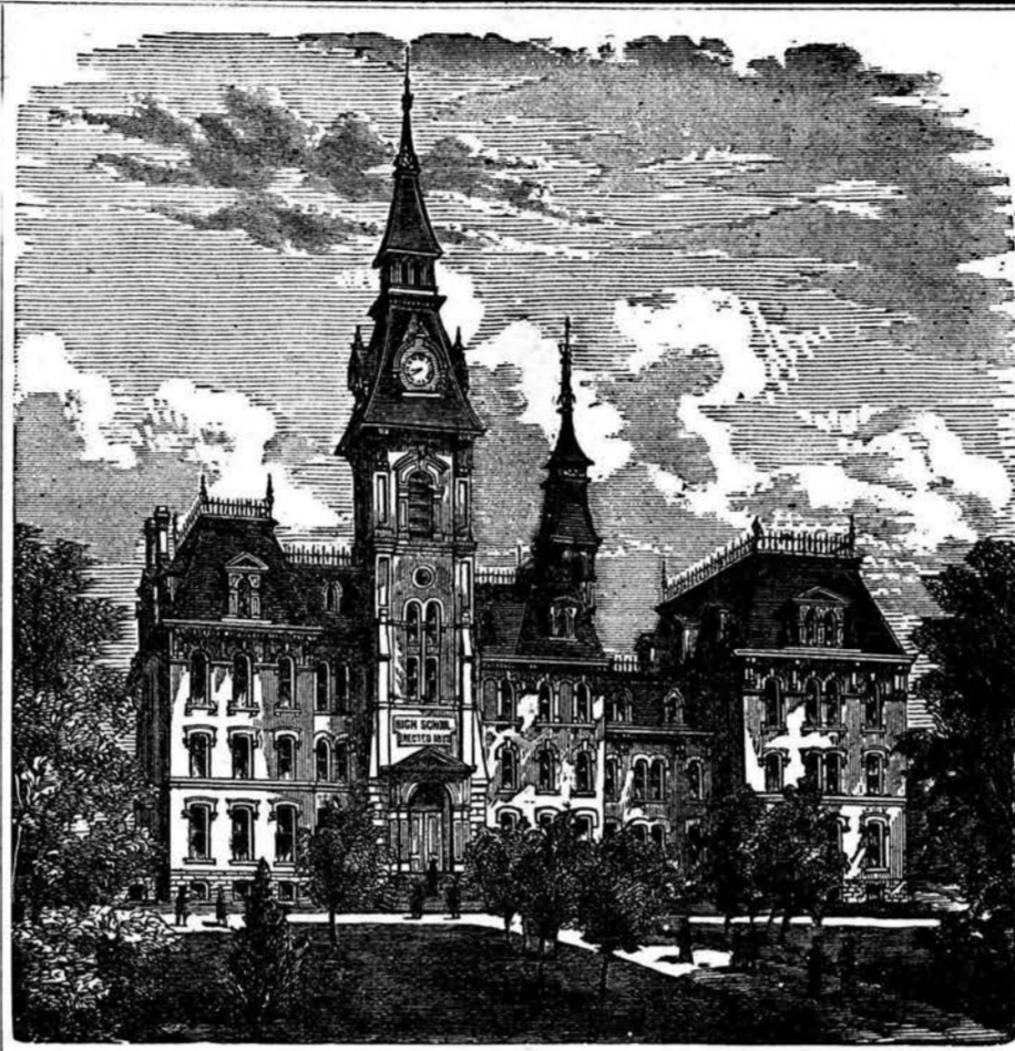
View of the Omaha High School Building.
