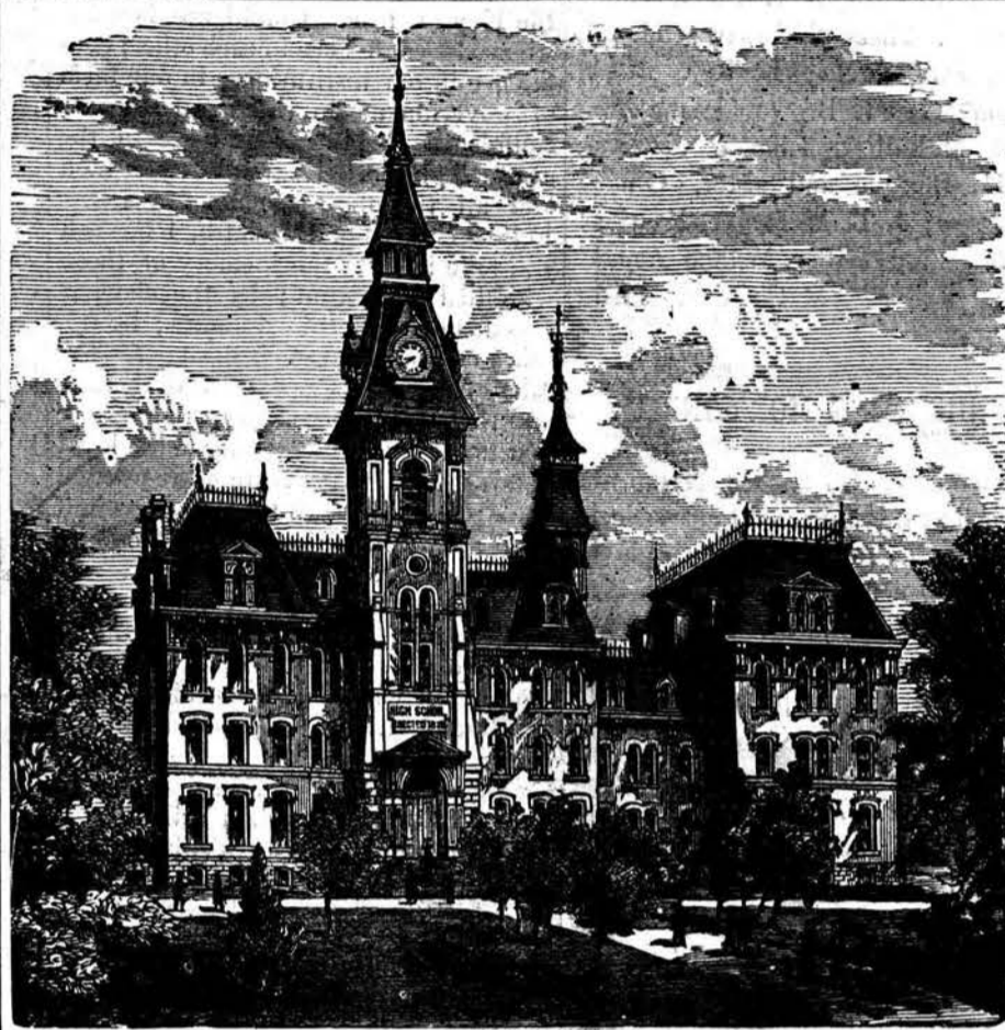
View of the Omaha High School Building.
