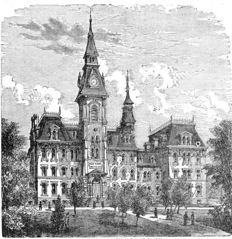
View of the Omaha High School Building.
