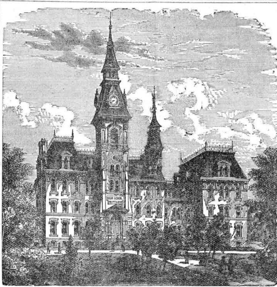
View of the Omaha High School Building.
