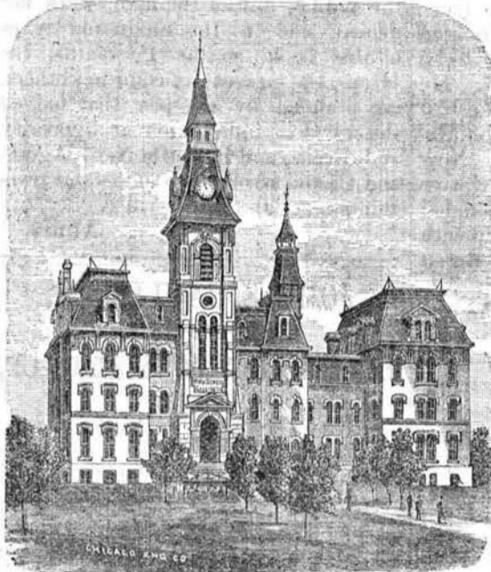
View of the Omaha High School Building.
