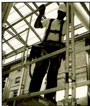
A construction worker stands on the scaffolding in the courtyard. The scaffolding was assembled so workers could reach the ceiling and work on the air conditioning socks. Photo by Clayton Lomneth.
