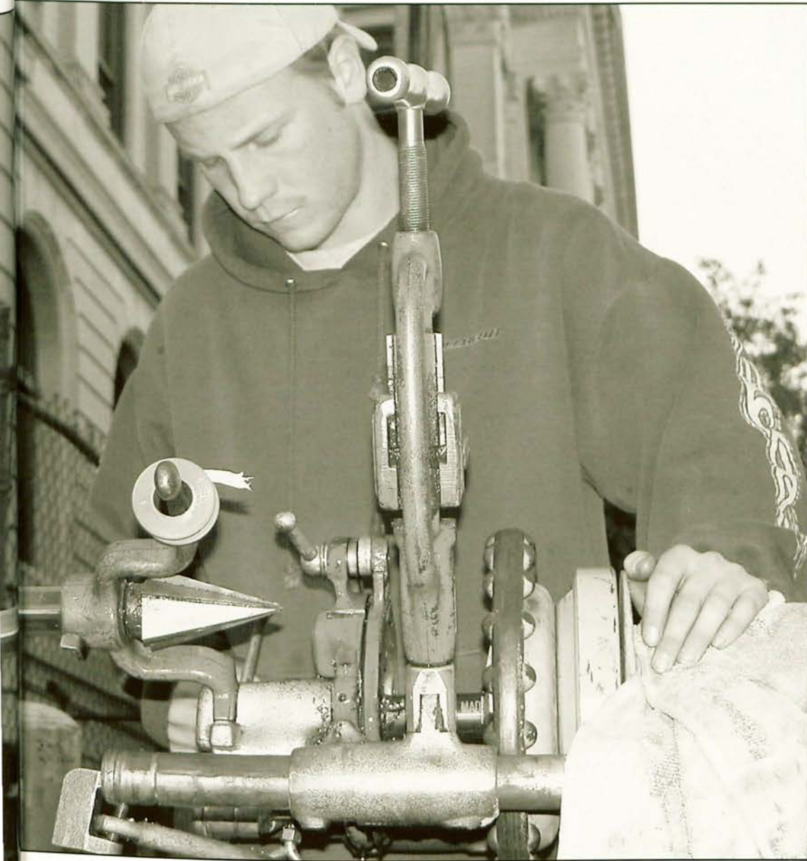
Left. Ryan Rinehart, from Total Fire Protection, works on cutting sprinkler piping to be installed in the auditorium.
