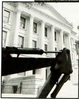
Above- A backhoe sits on the west side of the school in an enclosed area that blocked the primary walkway to the main entrance of the school. People had to walk across the turf to enter through the school's west side. Photo by Doug Meigs
