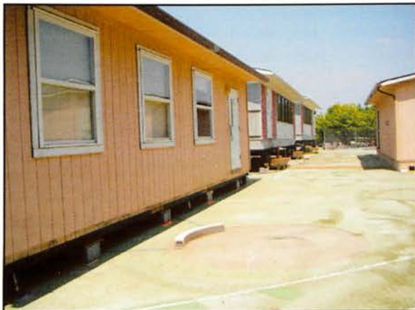
Left- The portables sit on cinder blocks on the turf in August, awaiting final installation. Photo by Kaitlin Jessing Batz
