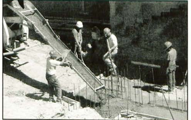
Above- Workers pour cement as part of the foundation for an addition. Photo by Kaitlin Jessing Butz
