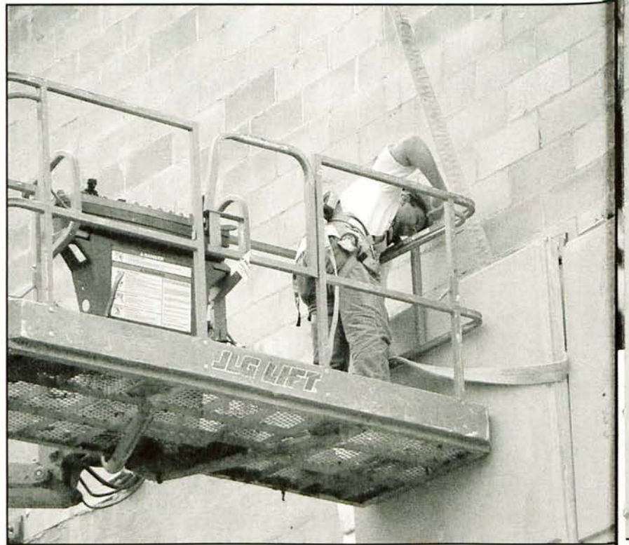
Above- A Hawkins Construction worker carefully pulls a slab off of the side of the building. Photo by Paula Salhani
