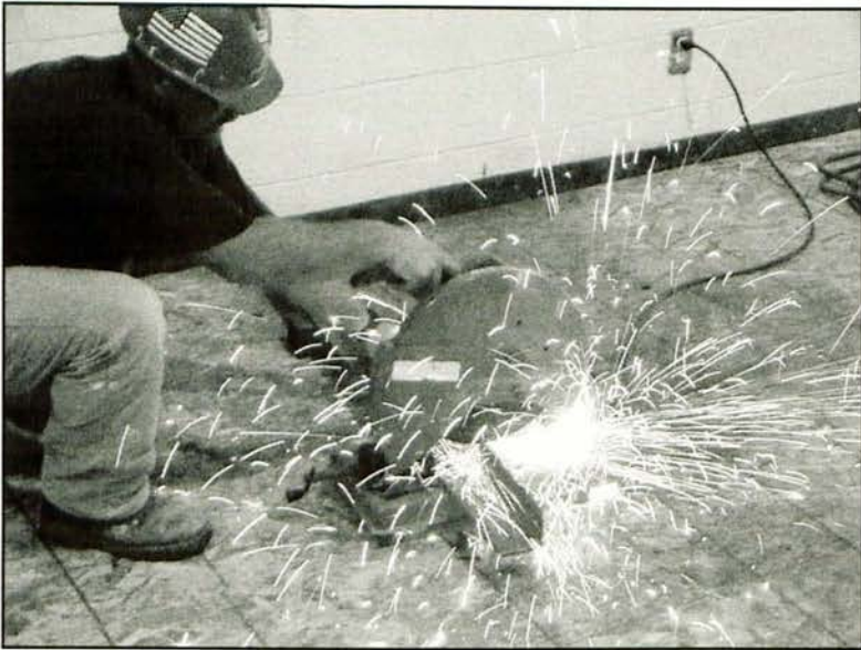
Above- Sparks fly as a Hawkins Construction worker cuts a piece of metal with an electric saw. Photo by Doug Meigs.
