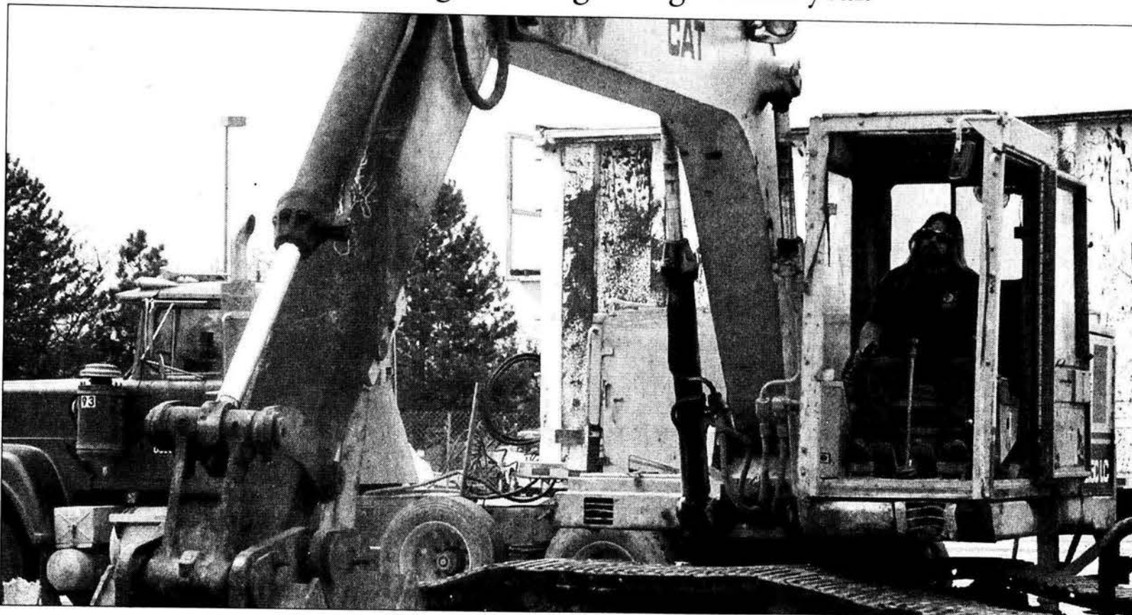
All photos by MICHAEL SMITH/THE REGISTER A construction worker operates a forklift while tearing up the turf to make room for the new portables. For more on coaches' and players' best memories of the Central field, see page 11.
