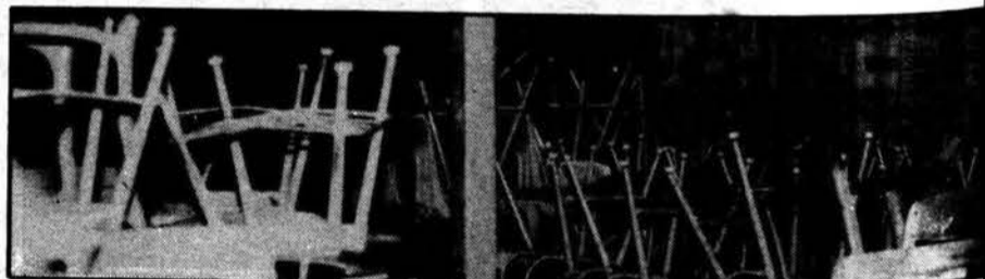
Now a bricked-in storage room for unused desks, this area used to be a low courtyard.
