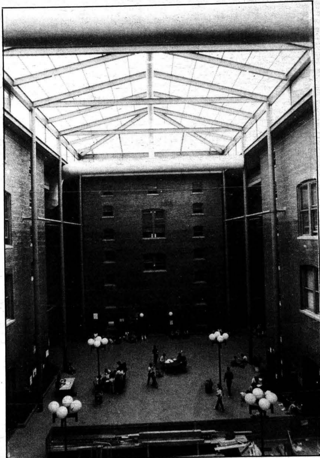
With the addition of a dome in 1981, the courtyard now provides a pseudo-outdoor atmosphere for students enjoying lunch. Pictured here are Centralites eating lunch during seventh hour with the construction worker's center evident in the foreground.
