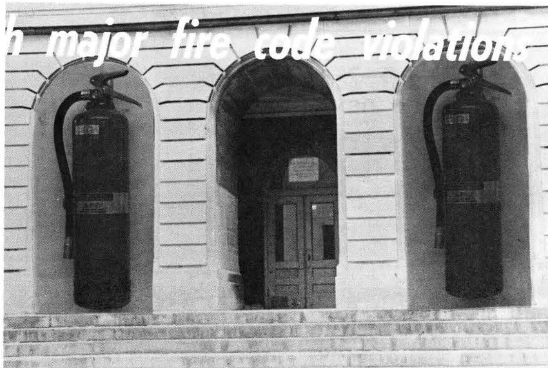
Possible "solutions" to fire code violations.
