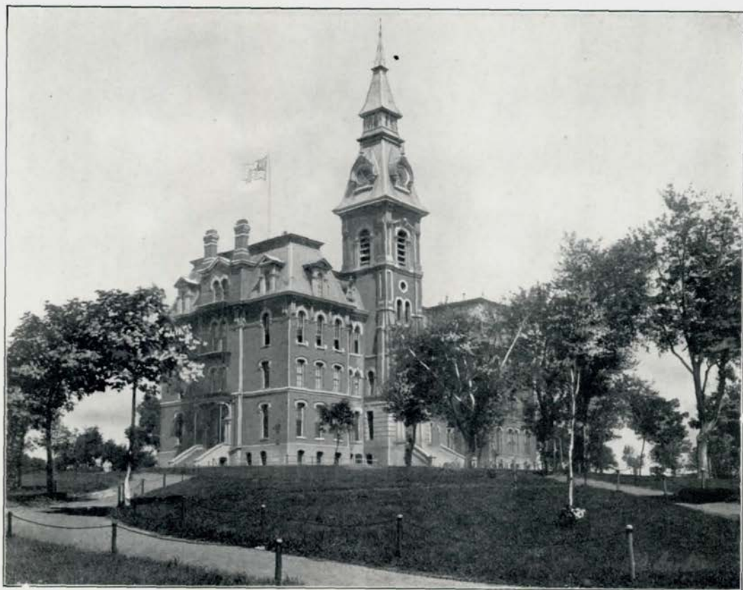
The Old High School Building.
