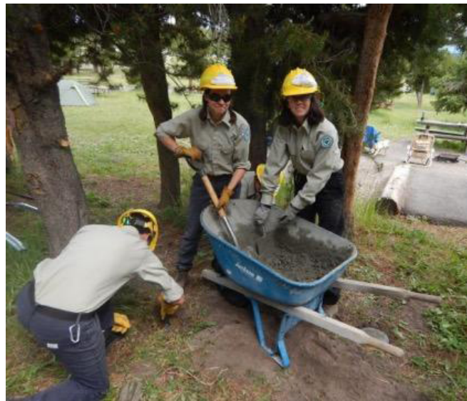
Left: The rangers and Hernandez mix cement for bear box forms
