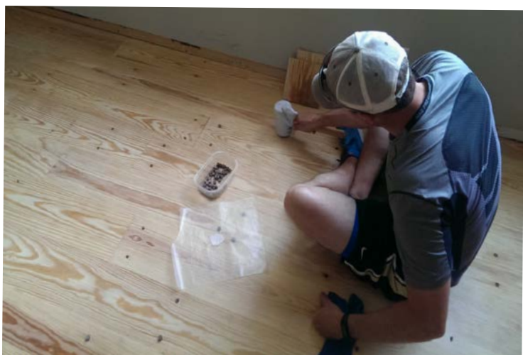
Step 5: Hamill fills holes in the newly installed floorboards.
